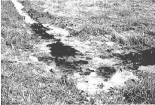
Failing sanitary sewer, causing upwelling of sewage through soil, and draining to gutter and then to storm drainage system.
